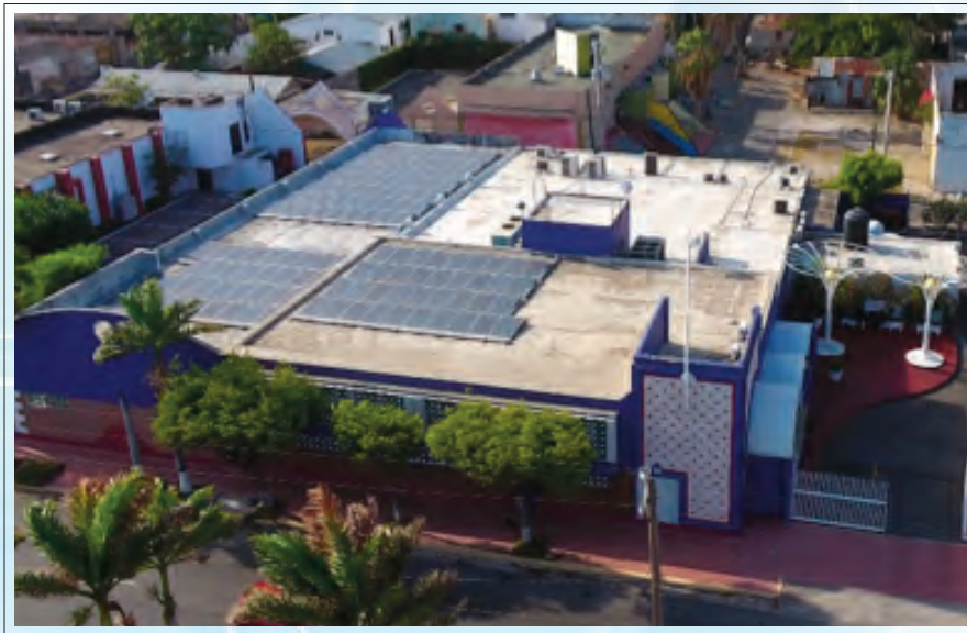
The Rooftop of the SMA displaying the Solar Panels which were installed in the second phase of its Grid-Tied Alternative Power Supply Project.
