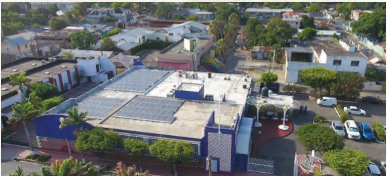
Figure 1 – A view of the SMA's main office building along Harbour Street, Kingston
