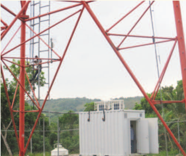
Maintenance being conducted at the Ocho Rios site.
